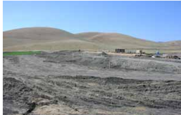
Grading for Gymnasium
