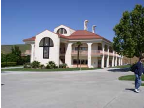
Existing Science Building 1800
