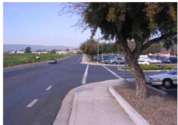
Existing Loop Road Image
