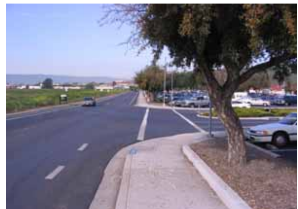
Existing Loop Road Image
