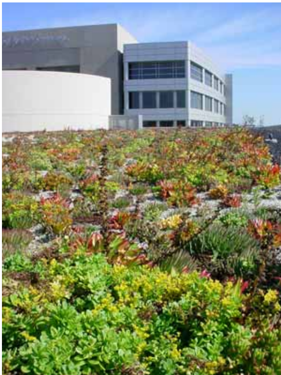
Green Roof To Reduce Heat Island Effect
