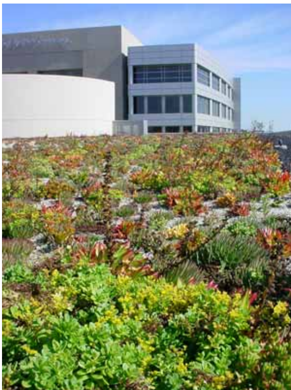
Green Roof To Reduce Heat Island Effect
