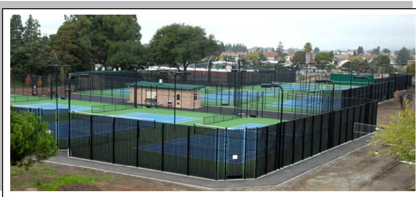
New Tennis Courts
