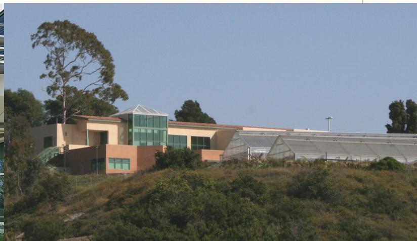
MiraCosta College Horticulture Complex, Oceanside, CA
