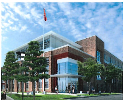
WEST CONTRA COSTA UNIFIED SCHOOL DISTRICT PINOLE VALLEY HIGH SCHOOL, Pinole, CA
