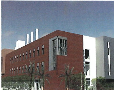
CONTRA COSTA COMMUNITY COLLEGE SCIENCE BUILDING 1 & 2 San Pablo, California
