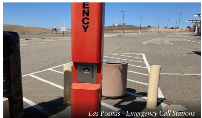
Las Positas - Building 1600 – Architecture Barrier Project
