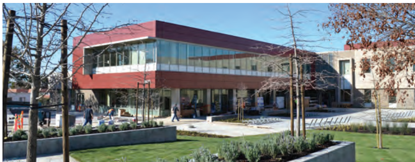
Las Positas College, Student Services and Administrative Building
