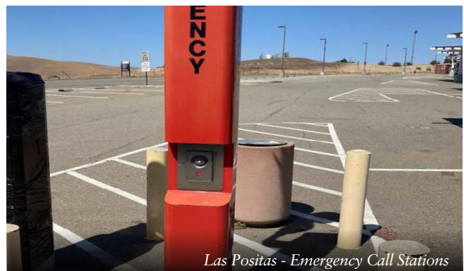
Las Positas - Building 1600 – Architecture Barrier Project
