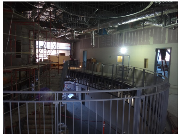
Lobby Stairs at Second Floor
