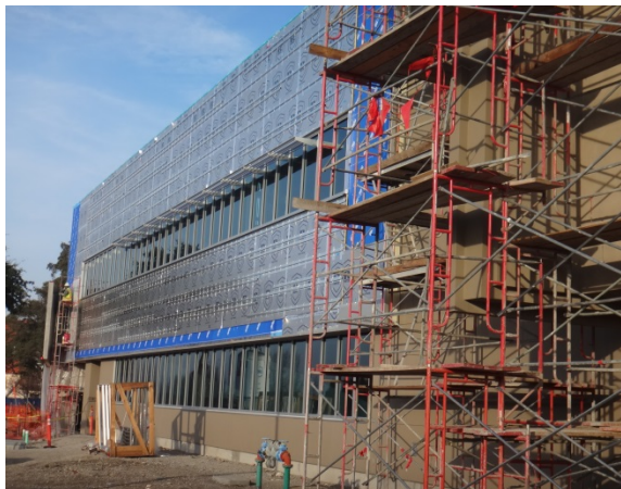
East Building View
