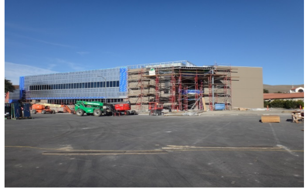
East Building View
