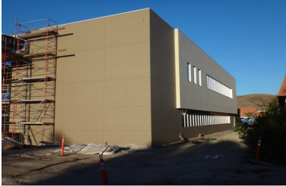
North East Building Corner
